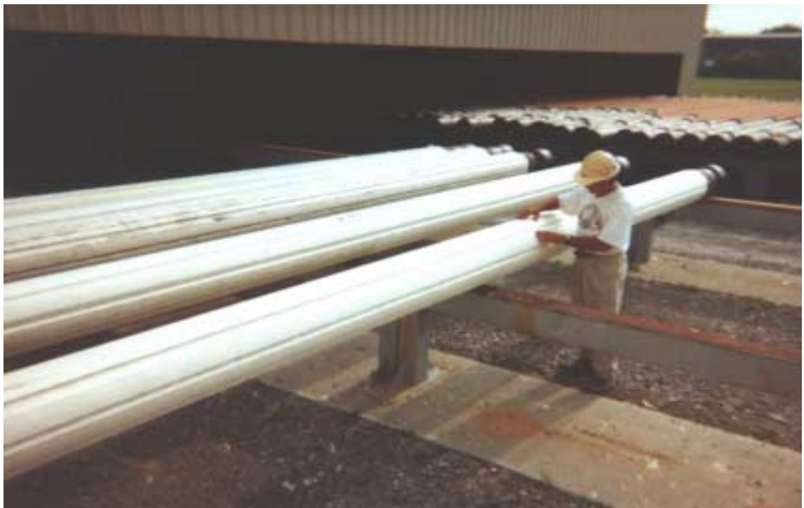
Figure 8 FINISHED JOINTS BEING INSPECTED
